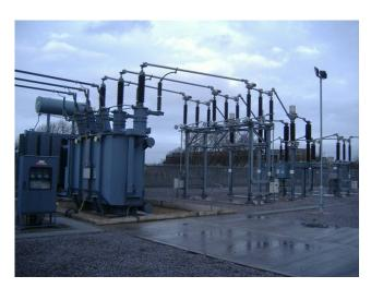
132kV Grid Substation showing main power conductors at high level but control circuits located in cubicles at lower level
