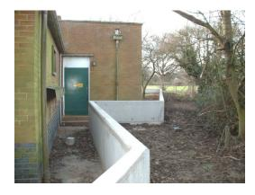
2 Construction of a waterproof wall within the site to protect critical assets. This option may be adopted where only specific assets are at risk and may be used in conjunction with option 3. Any of the following measures may be used where the flood height is not great, usually 300mm or less:
