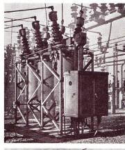
66-kV on Type 0W 407 circuit-breakers at Iver, Buckinghamshire.
