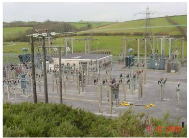
132kV Grid Substation showing 132kV terminal tower (pylon) and start of 33kV wood pole overhead line.
