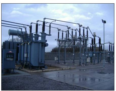
Photograph 3 - 132kV Grid Transformer and circuit breakers in service in the UK
