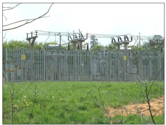
Photograph 6 - Primary Substation showing equipment operating at 33kV and 11k
