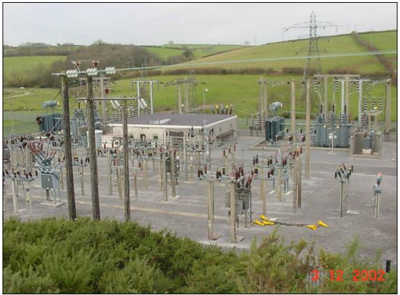
Photograph 5 - 132kV Grid Substation showing 132kV terminal tower (pylon) and start of 33kV wood pole overhead line
