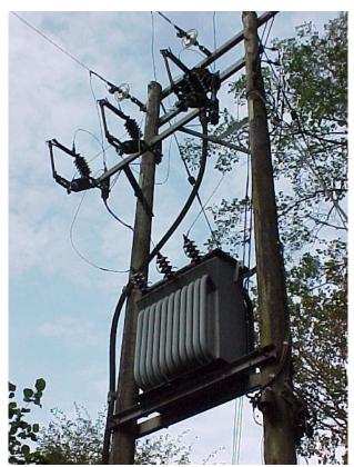
A pole mounted distribution transformer with external cooling tubes.
