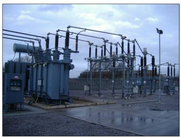
Photograph 8 - 132kV Grid Substation showing main power conductors at high level but control circuits located in cubicles at lower level
