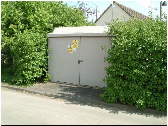
Photograph 7 - Distribution Substation with equipment operating at 11kV and 400/230 volts
