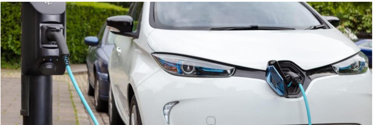
Figure 6: example of lamp-post public charging point, intended to reduce road-side clutter
